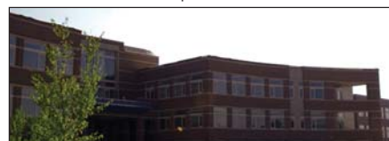
EB2, the new Computer Science and Electrical and Computer Engineering Building, which opened in the Fall 2005 semester
