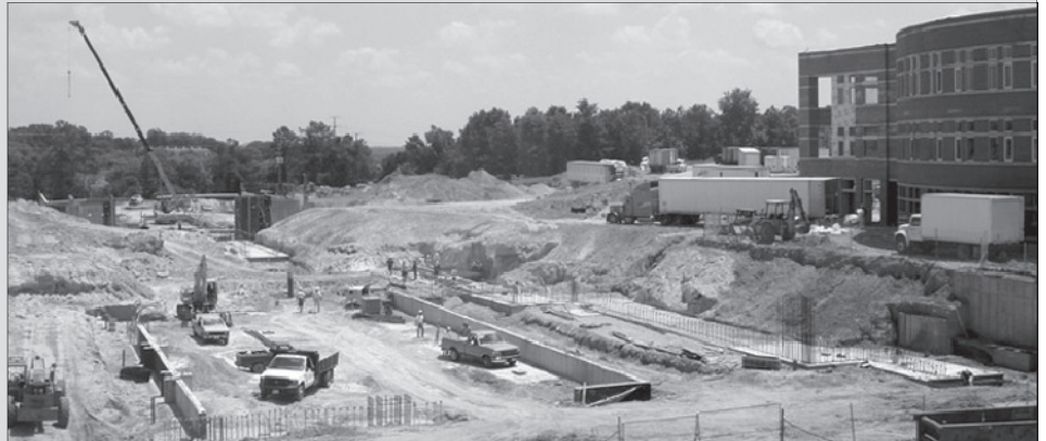
Construction site photo May 11, 2004. More photos and details online at http://www.csc.ncsu.edu/departments/facilities/newbldg_info.php .
